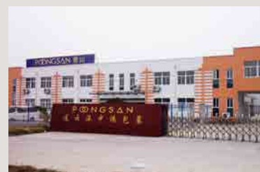
LOCATION : Dapu Industrial Park, Lianyungang, China PRODUCTS : Copper and copper alloy sheets and strips, brass rods, and stainless steel strips
